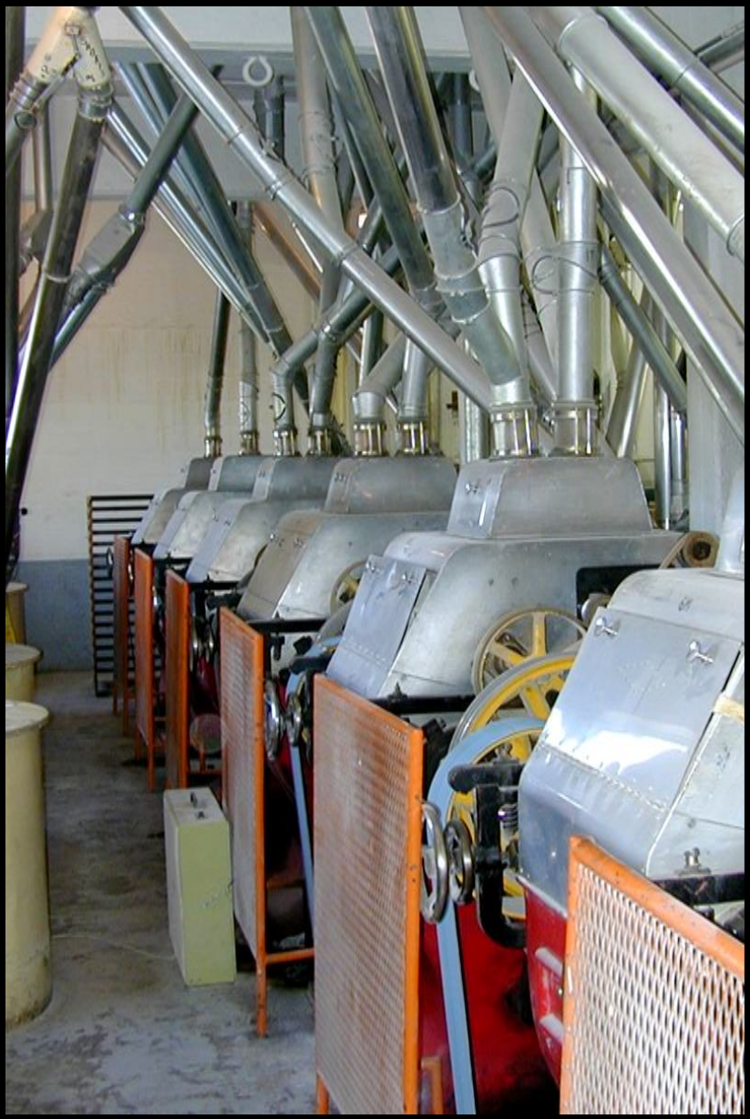
Before Structural Treatment
