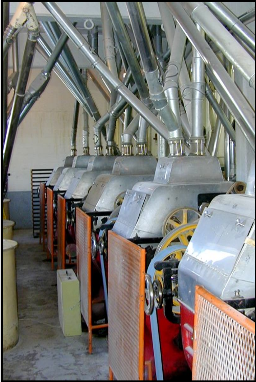
After Structural Treatment
