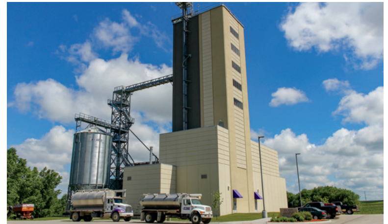
O.H. Kruse Feed Technology Innovation Center – a modern feed mill used for teaching feed production, pet food development, grain handling, and featuring an embedded BSL-2 research facility
