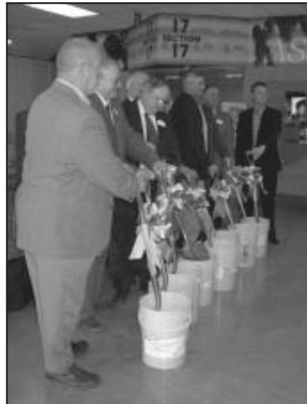
Members of the Kansas Wheat Commission symbolically break ground for the new IGP Executive Conference Center.
